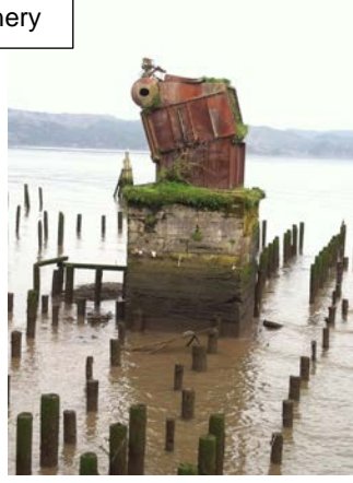
Former White Star Cannery adjacent to subject site; and existing remains of the cannery including the boiler, pilings, and ballast rocks.
