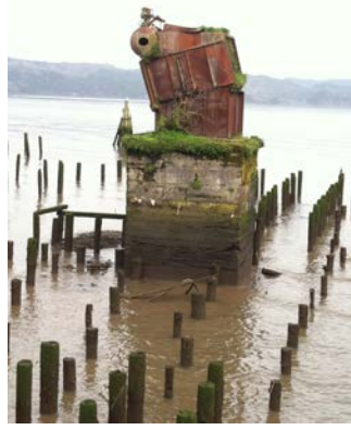
Former White Star Cannery adjacent to subject site; and existing remains of the cannery including the boiler, pilings, and ballast rocks.
